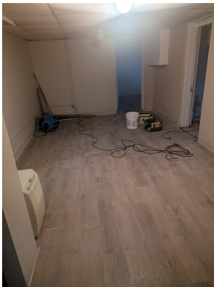
Recently remodeled basement adjacent to a full bathroom, utility room and storage room.
