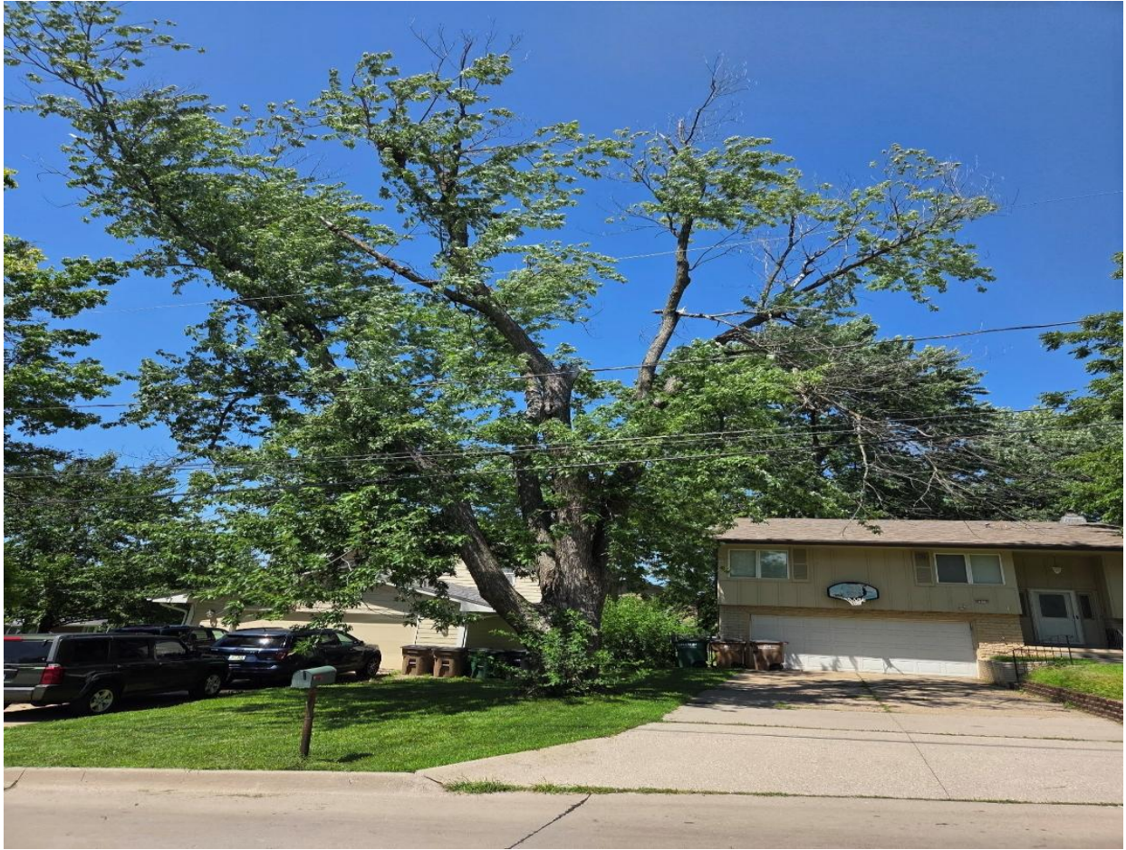
6315 Franklin: Dead branches overhanging driveway and house
