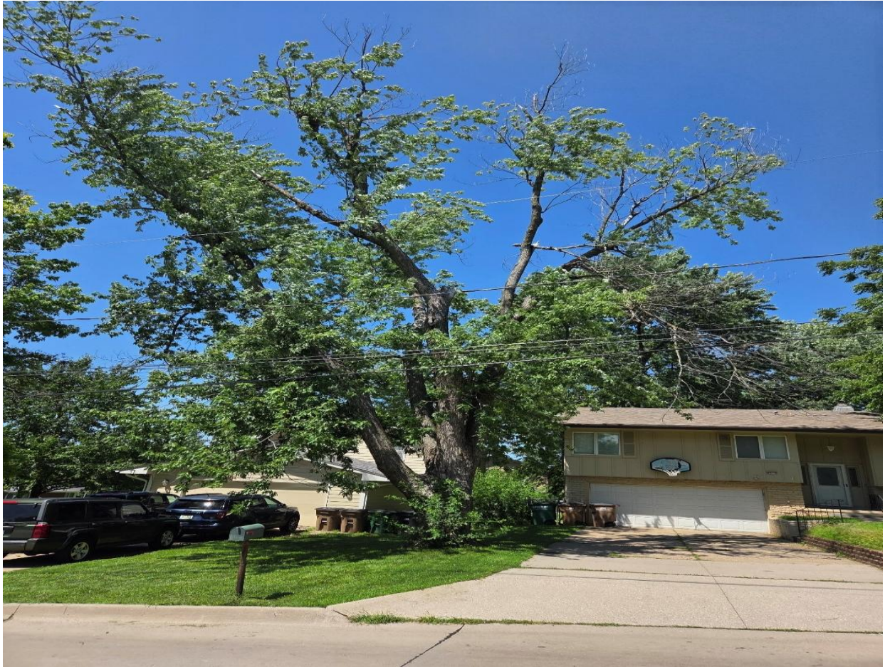
6315 Franklin: Dead branches overhanging driveway and house
