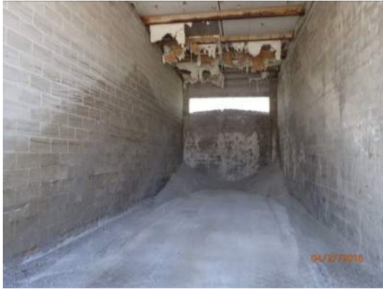
27, 28. Interior views of masonry distress and steel rusting
