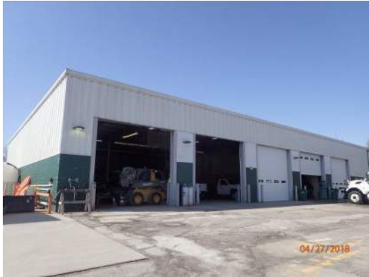
1. View from the northeast
