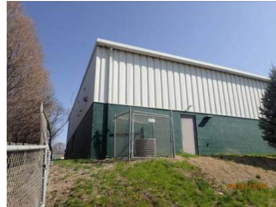
4. View from the southwest
