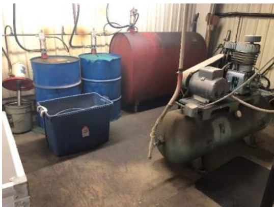
South end of mezzanine
