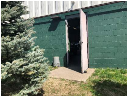
South elevation door
