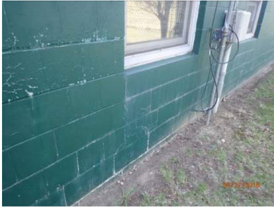
9, 10. Views of efflorescence
